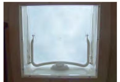
In order to open the skylight, press the release button to unlock the bracket and pull the bracket down. Then pull the bracket towards you to lock it into one of the three opening positions.
