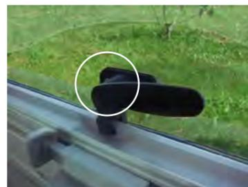
The windows can also remain open in a position for permanent ventilation by inserting the lever into the recess of the window lock.
